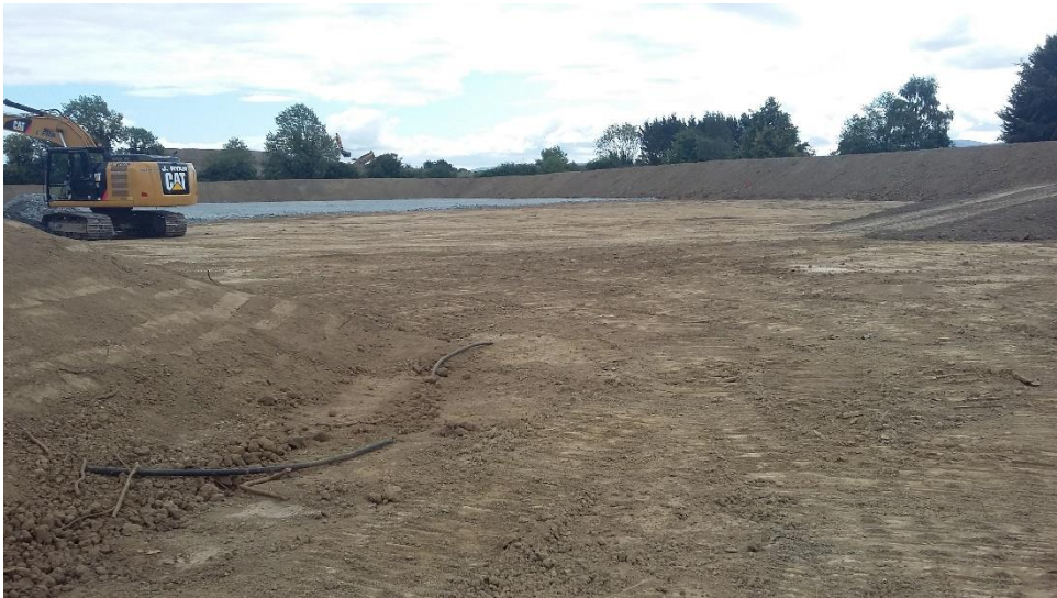
Figure 14.1 Levelling and laying with hard core of Ballybane Pitch & Putt Course
