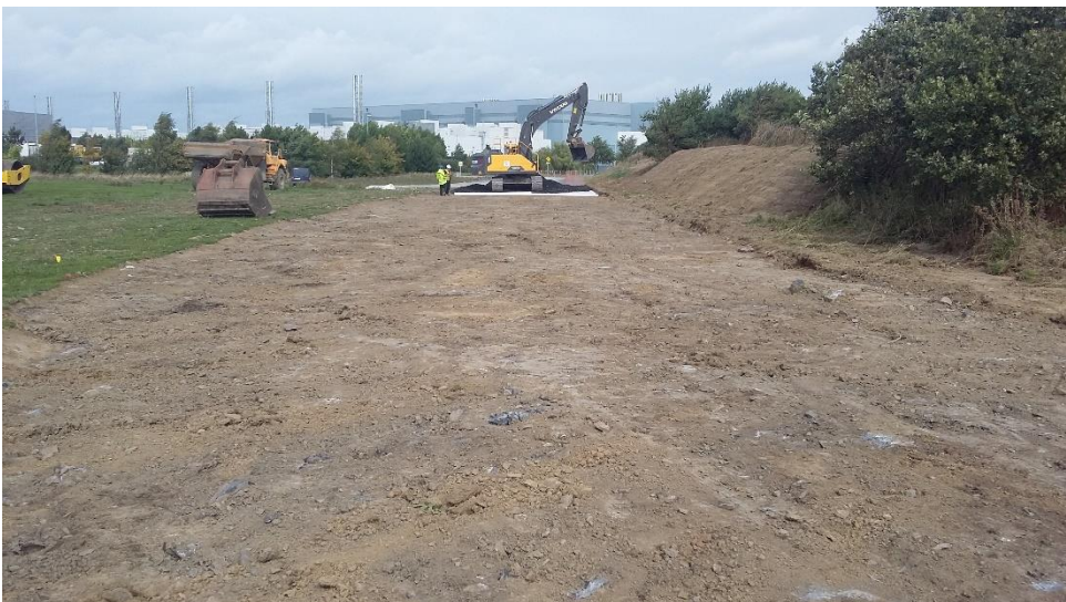
Figure 14. 3 Excavation of haul road in 'triangle' area facing west.
