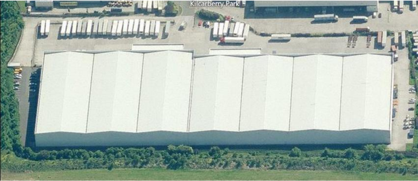
Figure 8.5: Commercial Façade Facing Grangecastle Site
