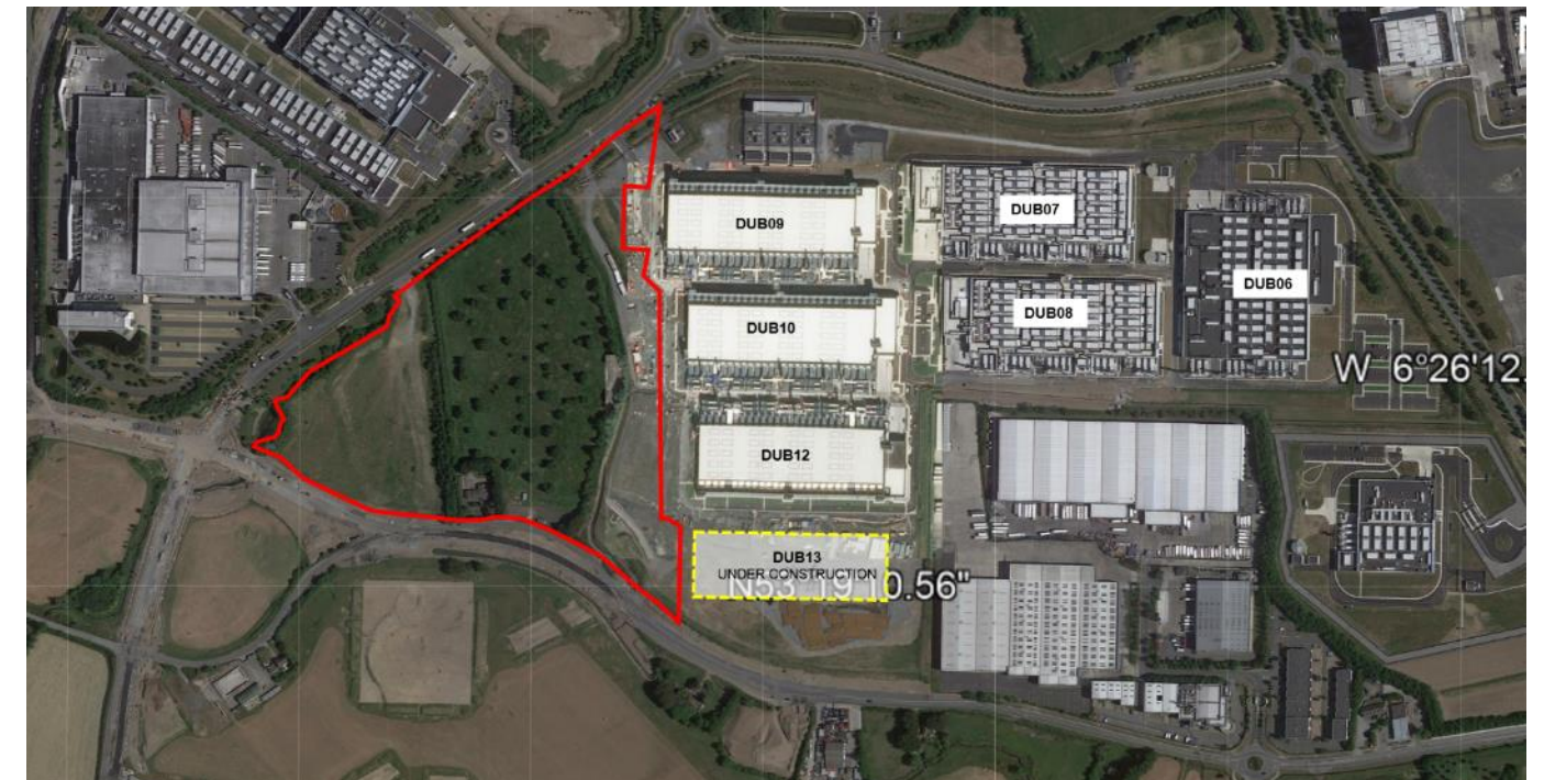
Figure 1.2 Adjoining MS Data Centres
